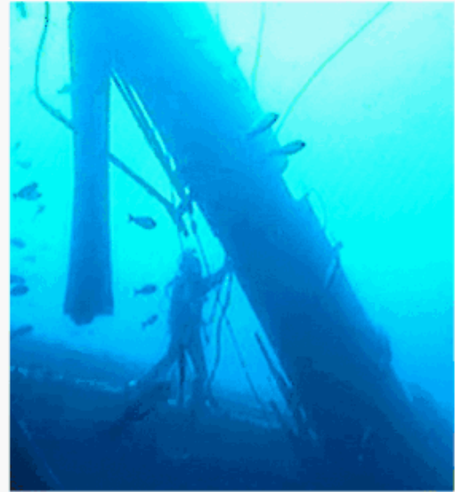
Underwater lighting system
